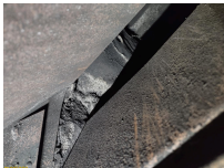
throat of chimney.jpg throat of chimney.jpg
