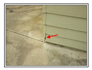
The siding seams are in need of caulking / sealing. Caulking / sealing of the siding seams should be included in a routine maintenance program.
