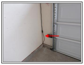
**Safety Reverses -** The garage doors are equipped with a safety reverse feature. During our inspection this feature did reverse when tested. Frequent testing is recommended to ensure proper operation.
