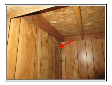
**Carbon Monoxide Detector** – Carbon Monoxide detectors are tested with the test button only. This type of test is not conclusive that the sensor is functional only that the test button feature is operational.
