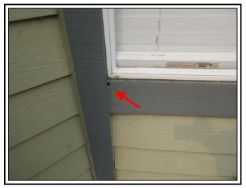
The wood trim is in need of caulking / sealing. Caulking / sealing of the wood trim and trim to siding contact should be included in a routine maintenance program.
