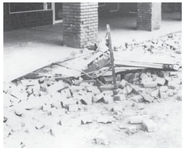
Figure 38 - The sign on this commercial building fell in the 1979 Imperial Earthquake.
