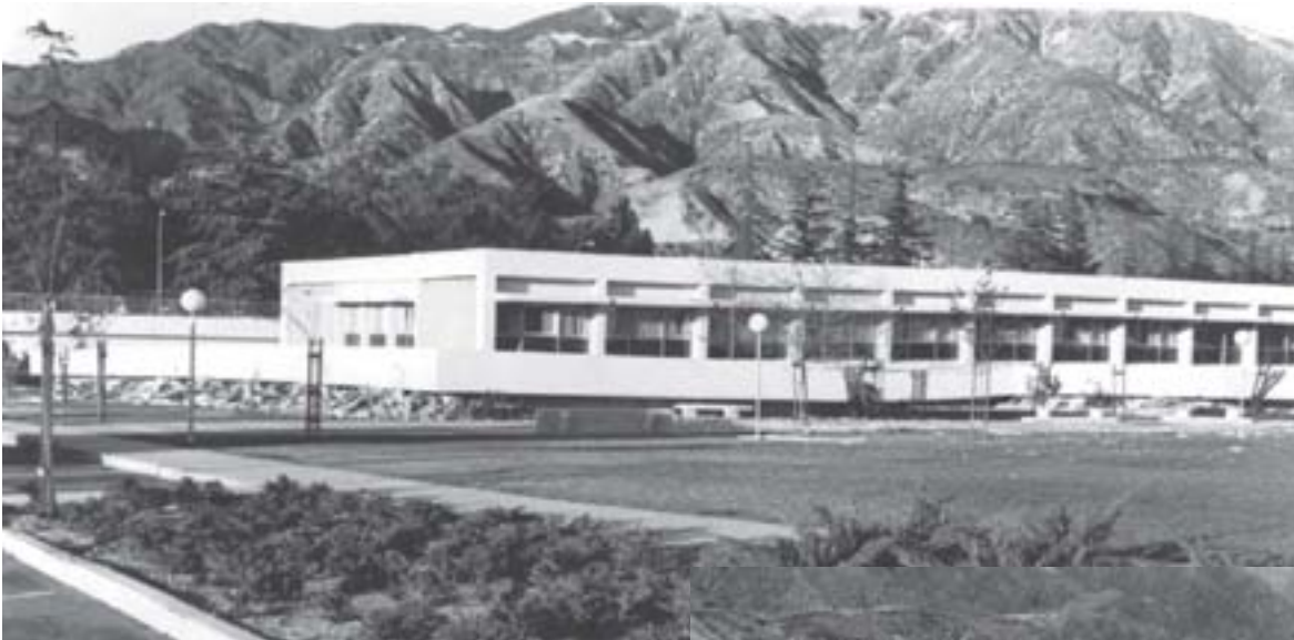
After the Earthquake
