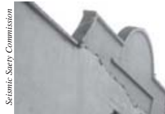
Figure 18 - Parapets. They are the tops of walls above the roof can fall off buildings like this one nearly did in Rio Dell during the 1992 Cape Mendocino Earthquake.
