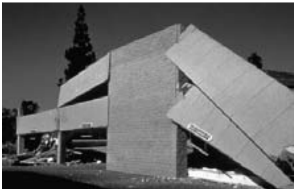
Figure 5 - Concrete Parking Structure Collapse.
