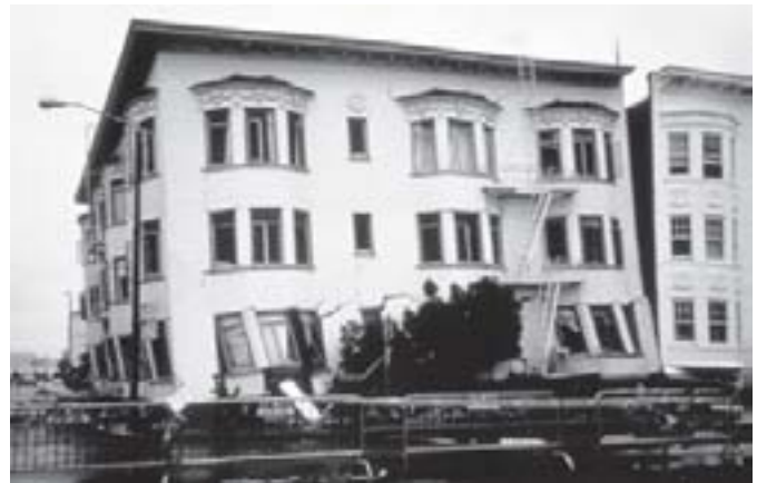
Figure 68 - Liquefaction caused differential settlement under this building and increased damage during the Loma Prieta Earthquake.
