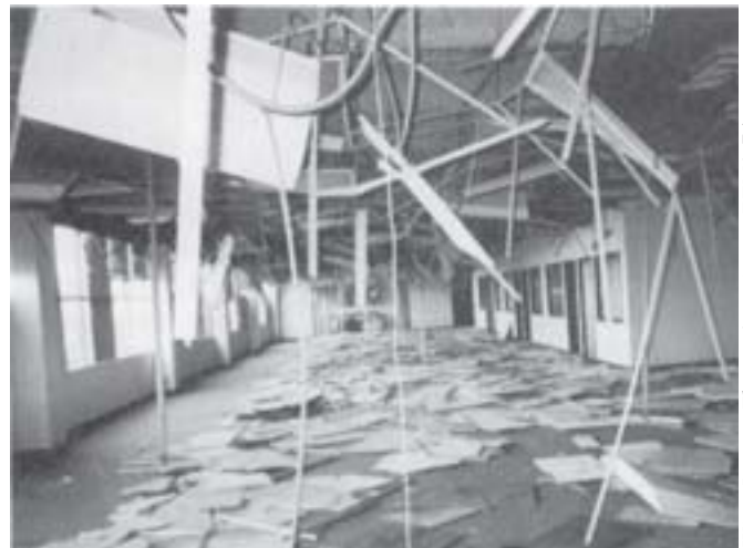
Figure 53 - This building sustained extensive interior nonstructural damage during the 1994 Northridge earthquake. Parts of the ceiling grid and tiles have fallen.
