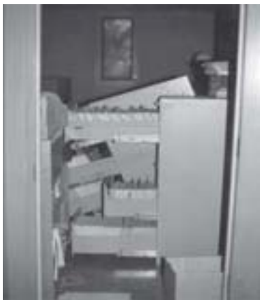
Figure 3 - File cabinet drawers can slide open and unbolted cabinets can topple during earthquakes.
