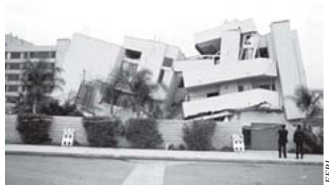
Figure 32 —This modern wood-frame apartment building had a central driveway. It collapsed inward over unbraced entrances to crush first-story parking during the 1994 Northridge earthquake.
