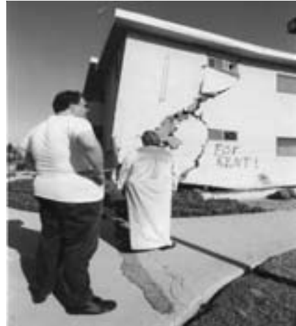
Figure 2 - Northridge Earthquake, Jan. 17, 1994. Collapse of the lower, soft story of this apartment rendered it uninhabitable.
