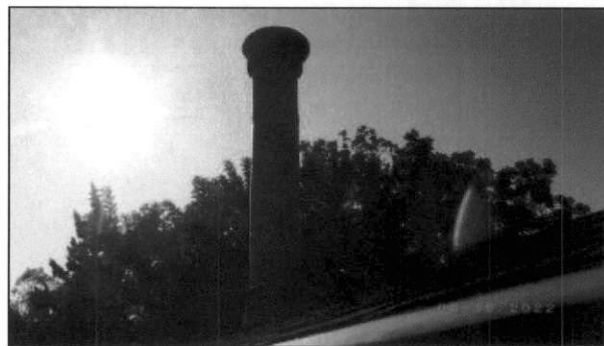
no view of flue interior
