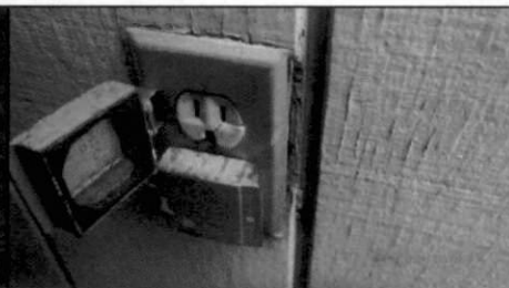
damaged outlet
