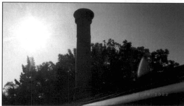
no view of flue interior
