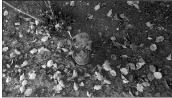
sewer clean out
