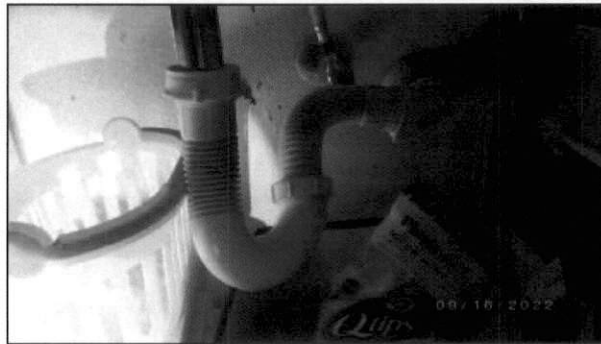
flex pipe used
