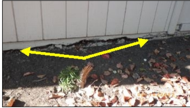
horizontal cracking
