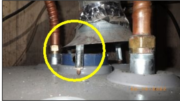
diconnected flue
