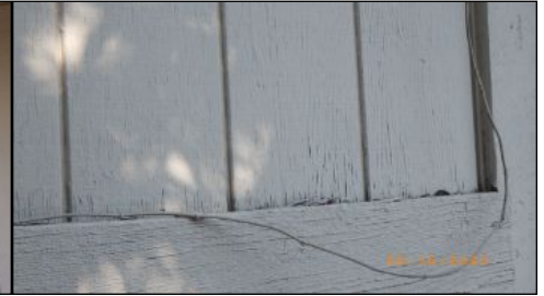
delaminated siding
